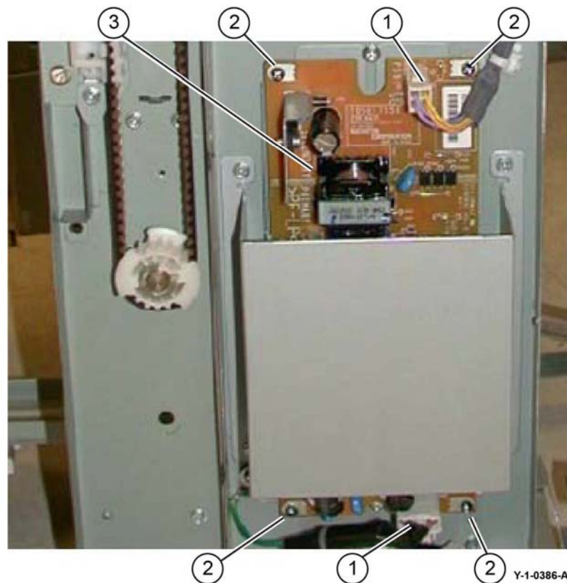
Figure 1 Finisher LVPS removal
